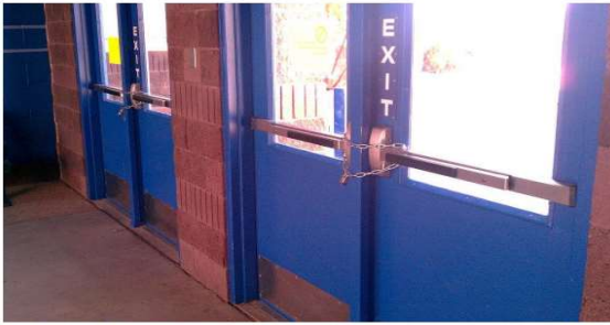
Fig. 1: Exit doors in a school, chained to provide security. This locking method does not meet IBC, IFC, or NFPA 101 requirements for free egress. Photo: Wayne Ficklin, Architect
