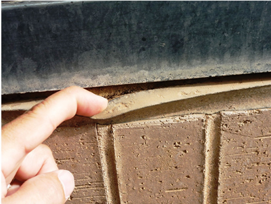
Window Sealant Failure
