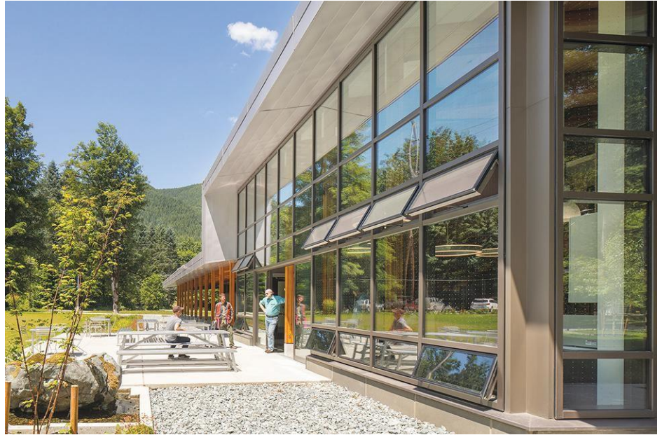
The City of Seattle’s Cedar River Municipal Watershed Headquarters located in North Bend, Washington, features bird-friendly glass with acid-etched designs so that birds can identify the glazing and avoid collision.
