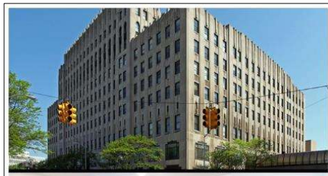
Albert Kahn Building – Detroit, MI
