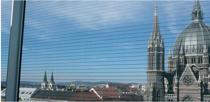
Horizontal black lines, 2 mm in diameter and with a 28 mm interval had very good Flight Tunnel test results – against all expectations. Where it is important to have the best possible visibility, in front of light backgrounds, this is an acceptable compromise.
