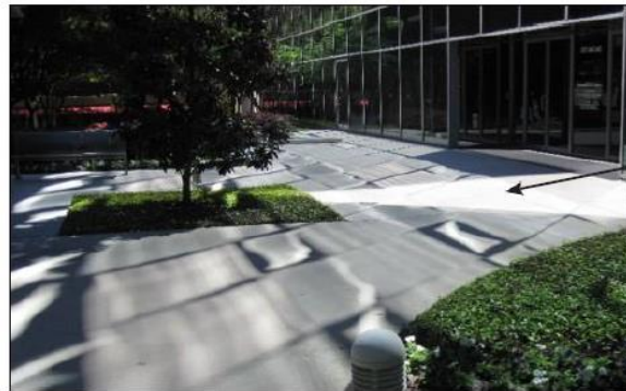
Figure 7: Reflection of light from insulating glass unit deflection
