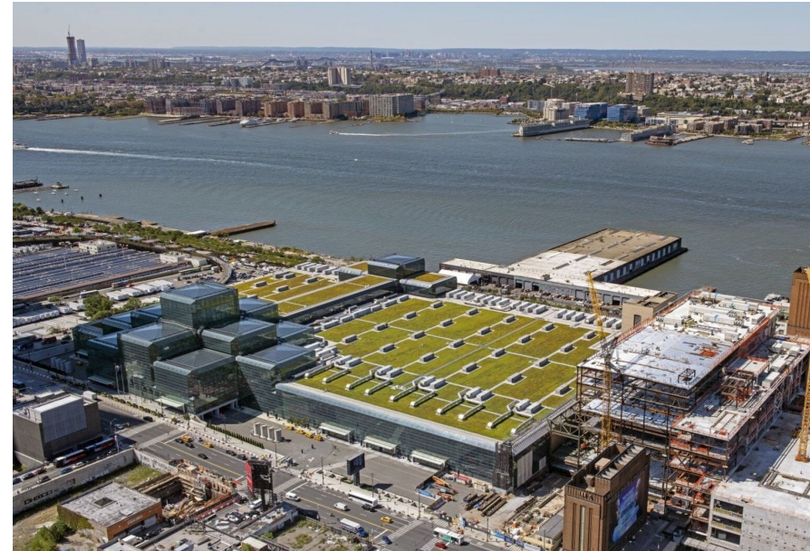
New York City's Javits Center, which was renovated with bird friendly glass in 2015, has reduced collisions by 90%.
